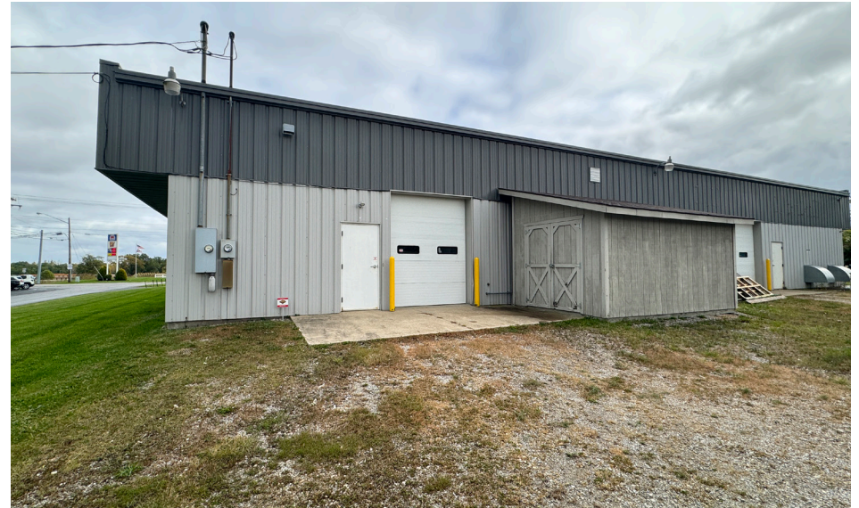
Rear Garage Door
